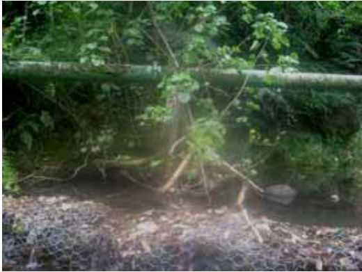
Stream crossing – wire mesh wall has constructed to protect the pipes
