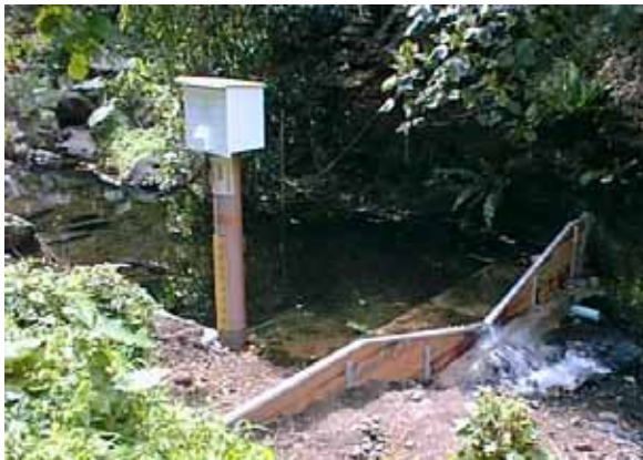
Water flow gauging station
