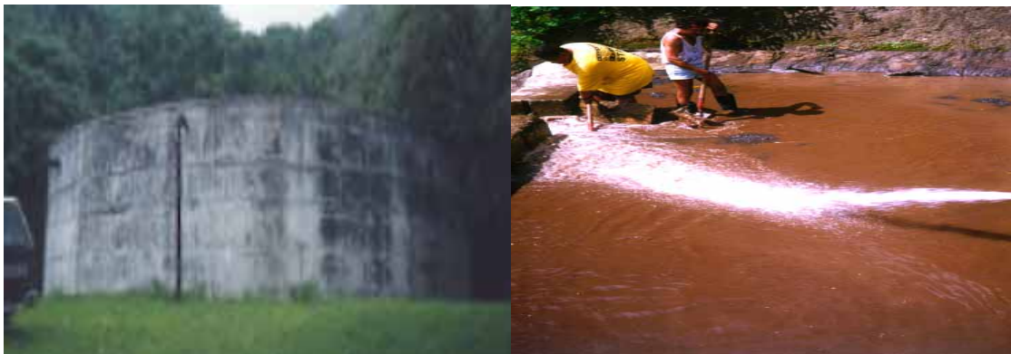
2.5 million L concrete tank at Takuvaine Intake cleaning after heavy rain and floods
