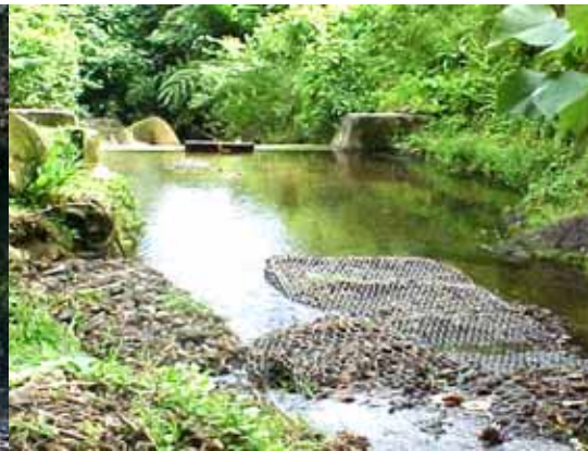
Wire mesh to cover the stones at intake
