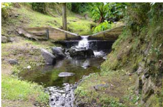
FIGURE 171. Water supply Intake in Rarotonga (Water Supply Master Plan for Rarotonga)
