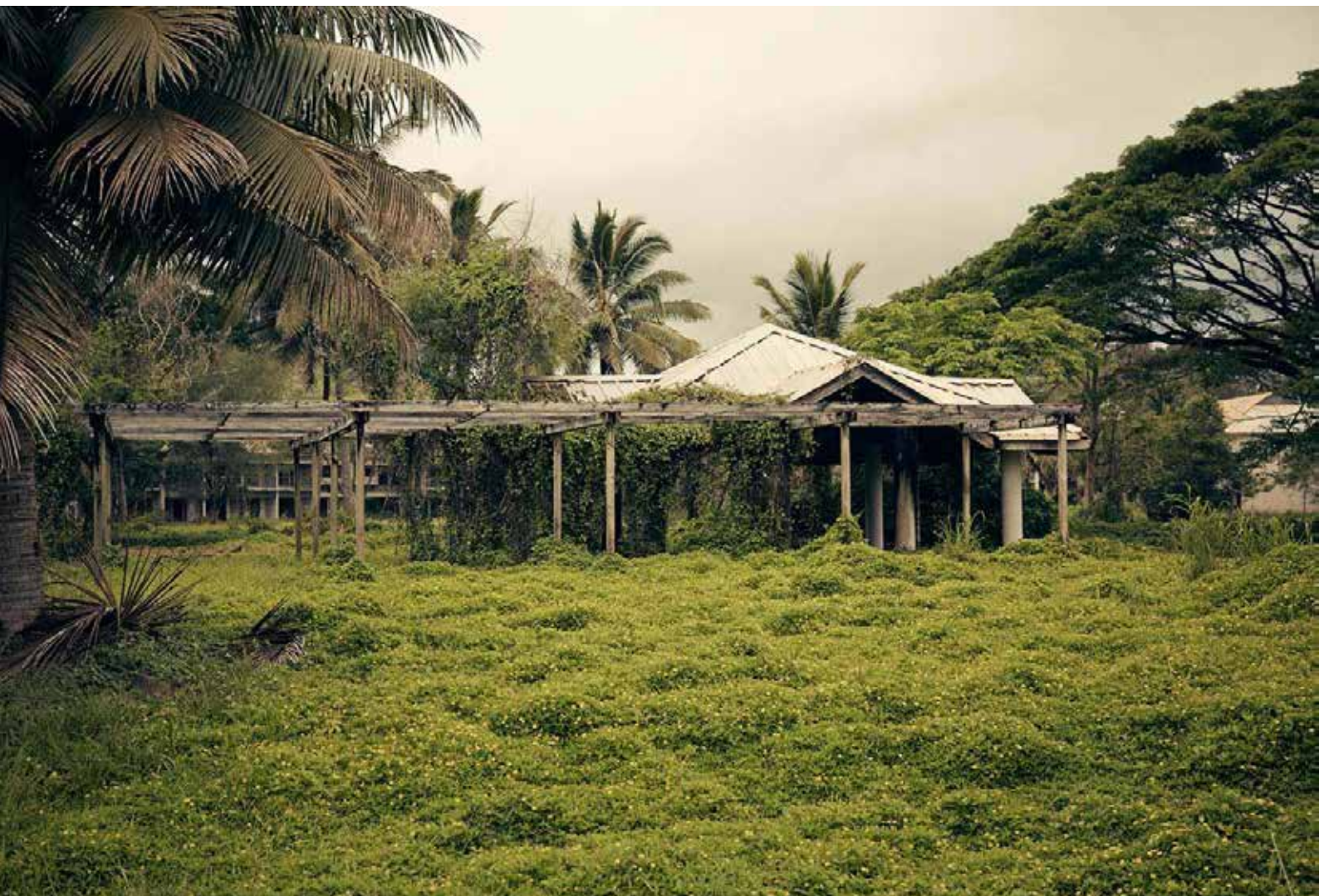
Ground and building covered with invasive plant species. (Olly Burn)
