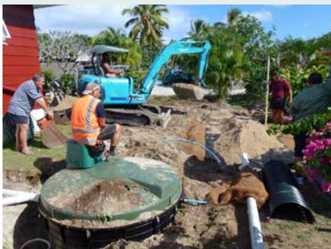
FIGURE 178. Muri/Avana Septic Upgrade Work, 2012. (WATSAN Website)
