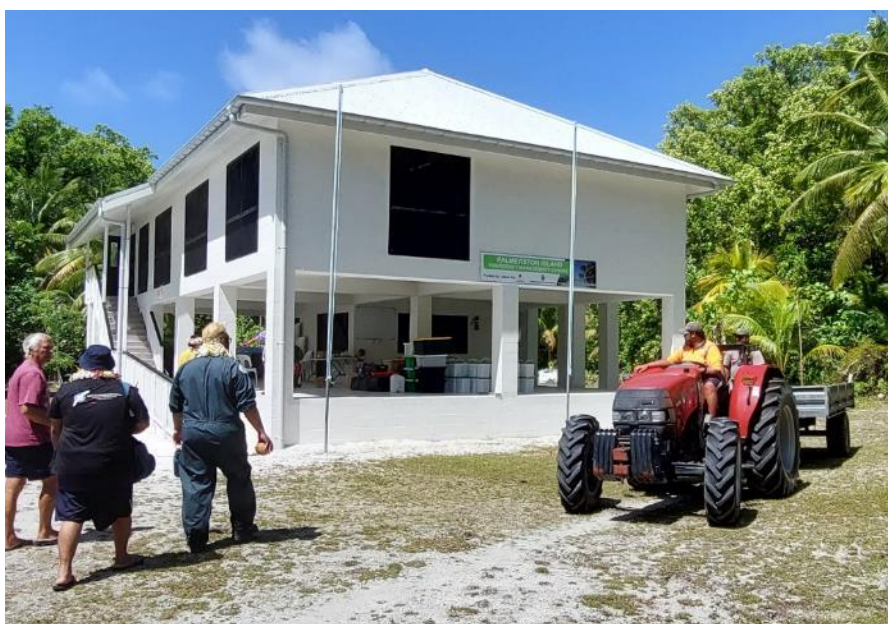
Figure 15: Emergency Management Center where the field team operations will be based from, Home Island
